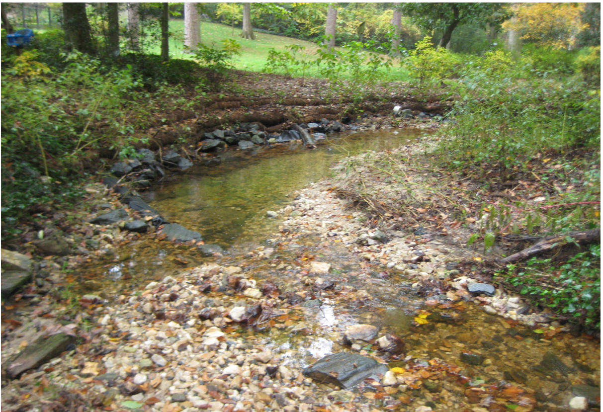
Coconut logs, live stakes, toe of slope protection and riparian restoration - Photograph courtesy of Register-Nelson Environmental Consultants.
